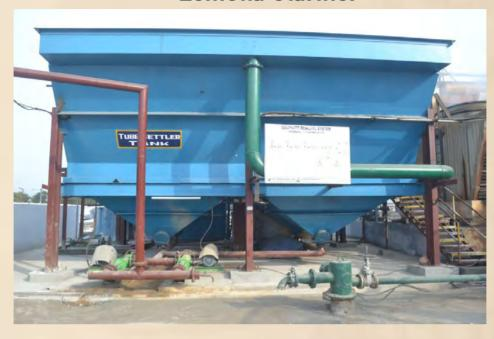
Tube Settlers are used in solid and liquid separation. It separates solid sludge from the wastewater. This process is purely based on gravitational. Media used in tubes settler increases the settling capacity. Multiple tubular channels are sloped at an angle of 60° and are adjacent to each other, which combine to form an increased effective settling area. pumped at a uniform rate to the plant.
