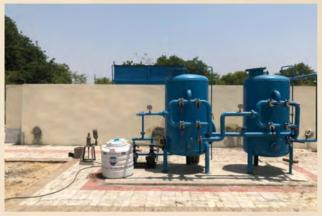
Activated Carbon Filter (ACF) works on the principle of adsorption. The filter media adsorbs or reacts with pollutant molecules, and then filtered water is drained out.
