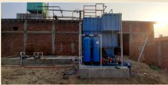
UY Trienviro designs, fabricates, installs and commissions different capacities of packaged sewage treatment plants as per the customer's requirements. These are suitable for rural areas, highway rest stops, hotels, restaurants and hospitals mainly where population is small or space is less or required plant capacity is small. The treatment scheme starts from bar screen, oil & grease trap, that flows to equalization tank which allows the flows
