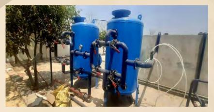
In Multi Grade Filter or Pressure Sand Filter, water is passed through multiple layers of filter media consisting of graded sand, pebbles and gravels layers. This arrangement captures contaminants in the media bed and filtered water passes into the discharge manifold at the bottom of the tanks. UY Trienviro provides MGF or PSF in MS and SS tanks using high-grade filter media and valves with epoxy coating. We also cater to special requirements.
