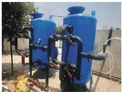
In Multi Grade Filter or Pressure Sand Filter, water is passed through multiple layers of filter media consisting of graded sand, pebbles and gravels layers. This arrangement captures contaminants in the media bed and filtered water passes into the discharge manifold at the bottom of the tanks. UY Trienviro provides MGF or PSF in MSEP and SS tanks using high-grade filter media and valves. We also cater to special requirements.
